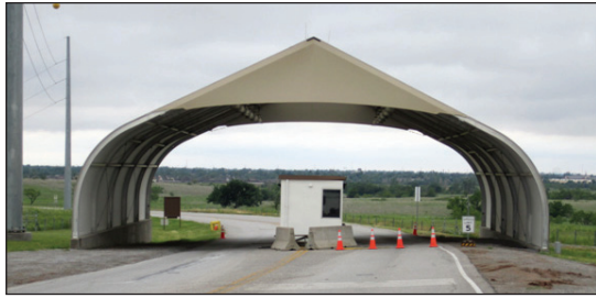
Figure. 1. Quonset hut-style tension fabric building at Fort Sill, Oklahoma, nested in by Scissor-tailed Flycatchers in 2010 and 2012.
