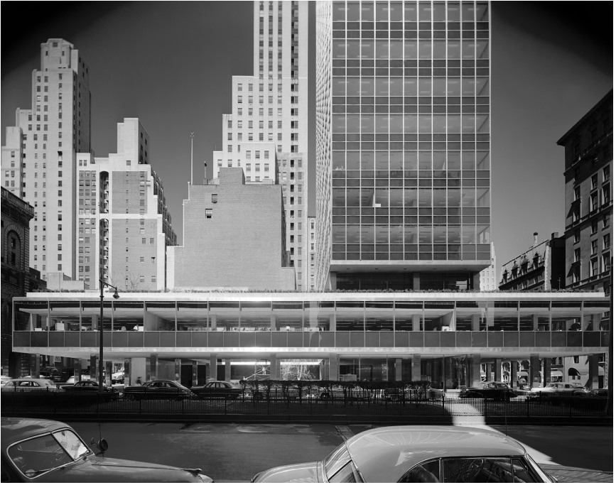
FIGURE 1: LEVER HOUSE (PRIOR TO RENOVATION)
