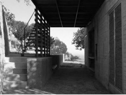
FIGURE 10: VIEW OF RETAINING WALL AND BUILDING SUGGESTING A KIND SPATIAL DIALOGUE BETWEEN THE TWO.
