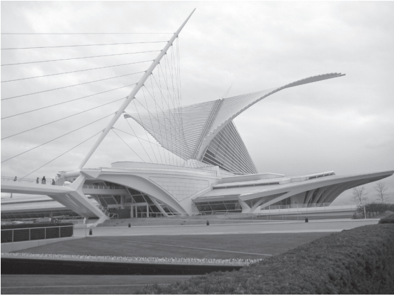
ANOTHER KIND OF ART AND SHOCK: CALATRAVA'S QUADRACCI PAVILION
