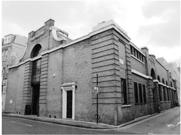
FIGURE 1. ISLINGTON TRANSFORMER STATION
