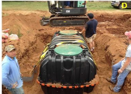
Appendix Figure 5. Pictures taken during the installation/construction of the Oklahoma Onsite Wastewater Training and Demonstration Facility. Initial layout of the trenches (A); graduate students laying-down the gravel (B); Installation of the tank donated by Clearstream (C) installation of the plastic composite tank donated by Infiltrator (D).
