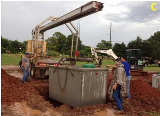
Appendix Figure 5. Pictures taken during the installation/construction of the Oklahoma Onsite Wastewater Training and Demonstration Facility. Initial layout of the trenches (A); graduate students laying-down the gravel (B); Installation of the tank donated by Clearstream (C) installation of the plastic composite tank donated by Infiltrator (D).
