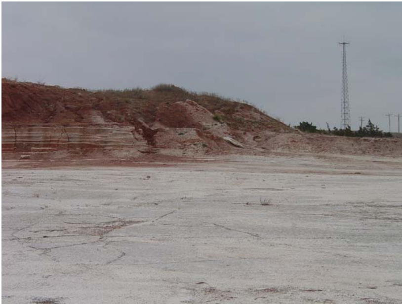
Figure 2. A view of the quarry floor looking east. The fractures in the quarry floor are visible in the foreground.
