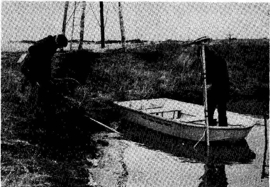
Figure 10. View of Wiring Burial
