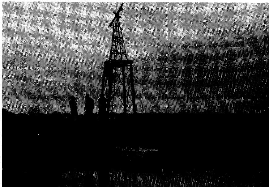
Figure 6. View of Completed Wind Generator Installation
