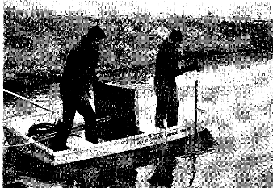
Figure 7. Installing Anchor Pole
