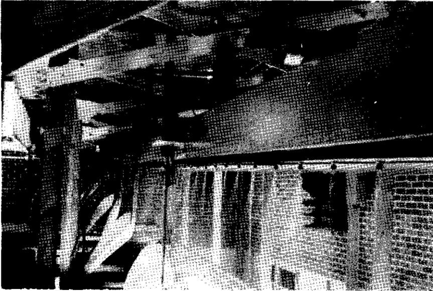
Cossett 1531 Type B pumps were used to withdraw water from a 9- by 5- by 5-foot sump. The intake for the sprinkler system had a 9-inch cubic steel frame covered with 16 mesh screen. Also a 20 mesh on-the-line strainer was placed in the sprinkler line to keep the nozzle heads and filters from clogging. Both systems had  $1\frac{1}{4}$  inch galvanized pipes running from the pumps to the upstream end of the channel. These pipes were supported by a large wooden frame.
