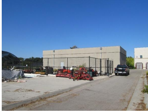
Figure 2. OSU-OKC Maintenance Shop (MS).
