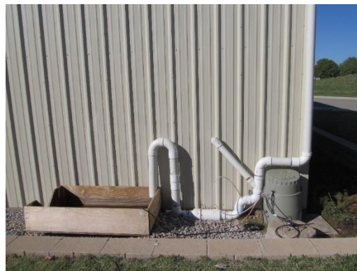
Figure 4. OSU-OKC HP downspout configuration.
