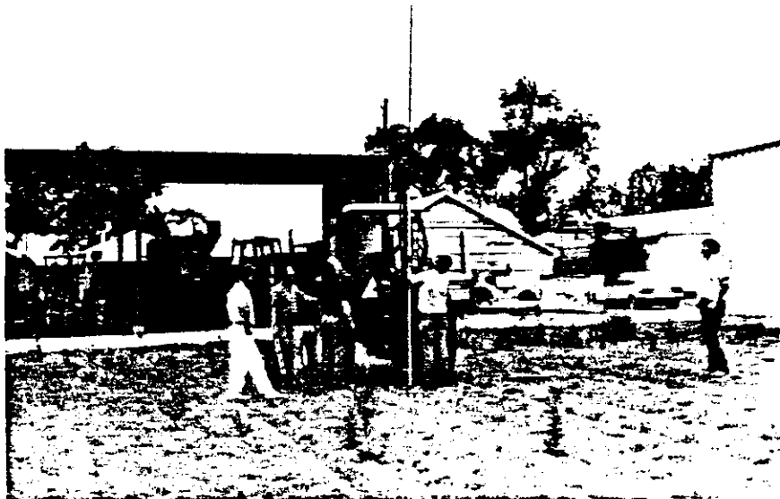
Figure 6. Ten foot joint of access tube being positioned on previously augered hole. Four researchers are being schooled in use of the device.
