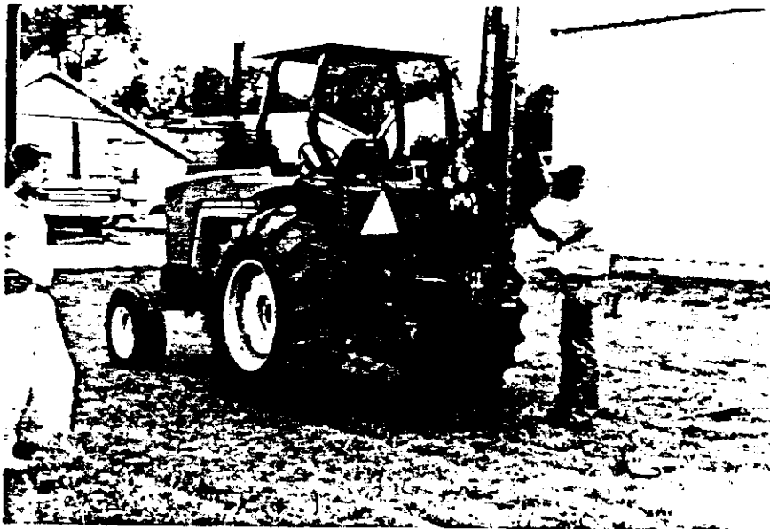
Figure 4. Tractor with tube installation device at the field site. The hole to accommodate ten foot access tube is being drilled.
