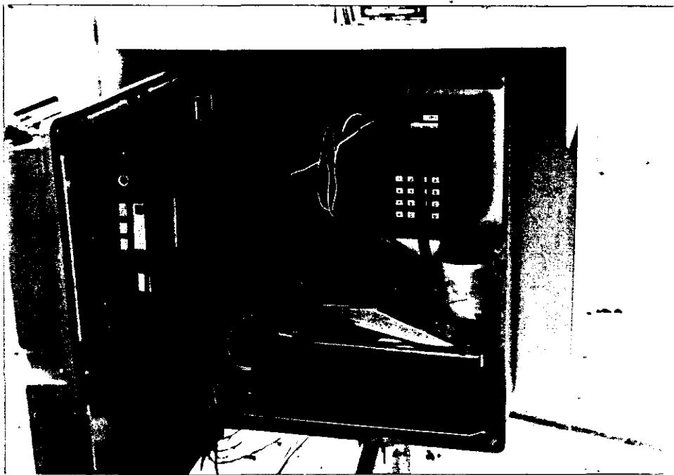
Figure 8. Weather data logger, printer, and cassette storage.
