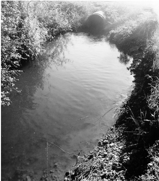
Figure 1. Study site in McCurtain County, Oklahoma. Note the drainage culvert at top of photograph.
